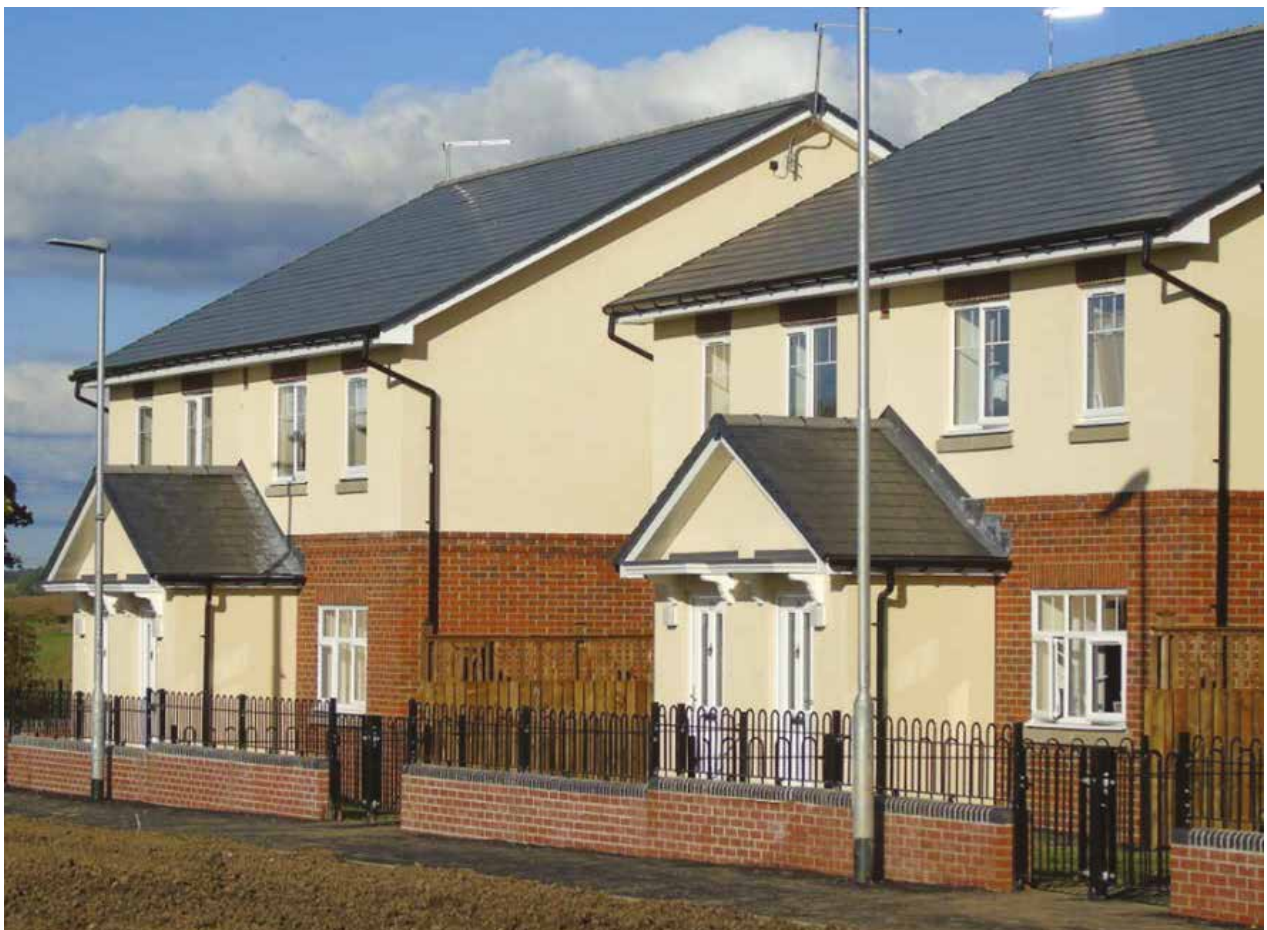
Example of new houses at Red Hall, Darlington
